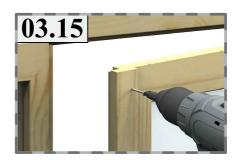
All windows are packed fully assembled. Window handles should always remain inside (03.12). Cover strips (if included in the assembly set of a window) should be fastened with screws (03.13-14). In the case of double windows opening to the outside, a connection strip should be installed which is fastened to the outside of the house (03.15). **NB! When installing the windows in the house, ensure they open on the correct side.**
